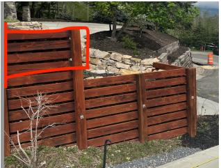
Picture 2: Retaining wall section higher than 4ft.
