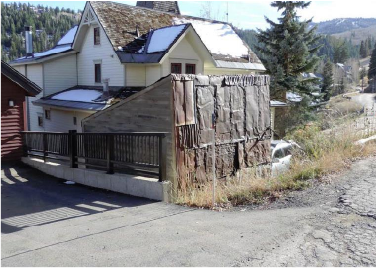
135 Sampson Avenue. Northwest oblique. November 2014.
