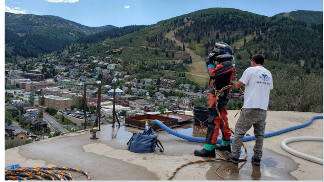
DIVER CONDUCTING ROUTINE WATER TANK CLEANING
