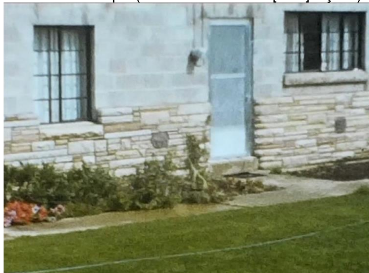
South façade (front half)
