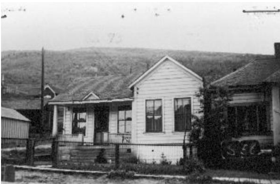
Figure 3: 1103 Woodside Avenue circ. 1940 tax photograph. Visible in this photograph is the single-car garage with its white-painted, board and batten siding and wood-shingled roof.
