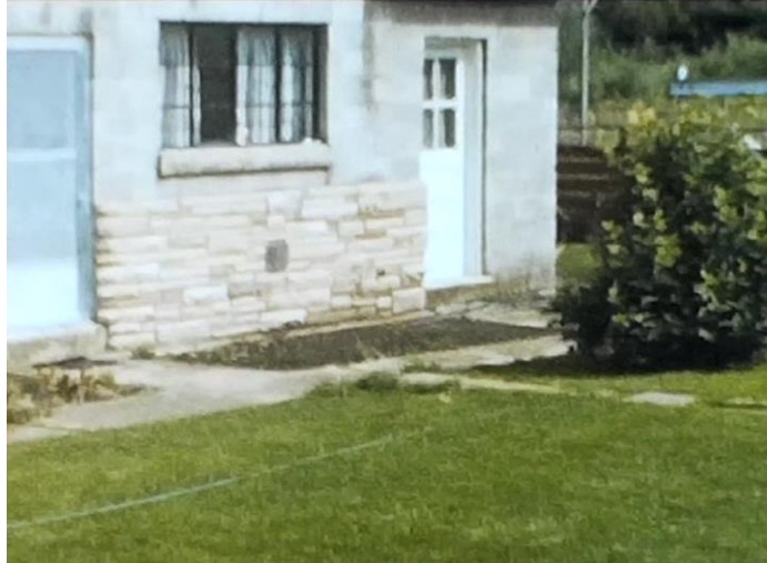
South façade (rear half)
