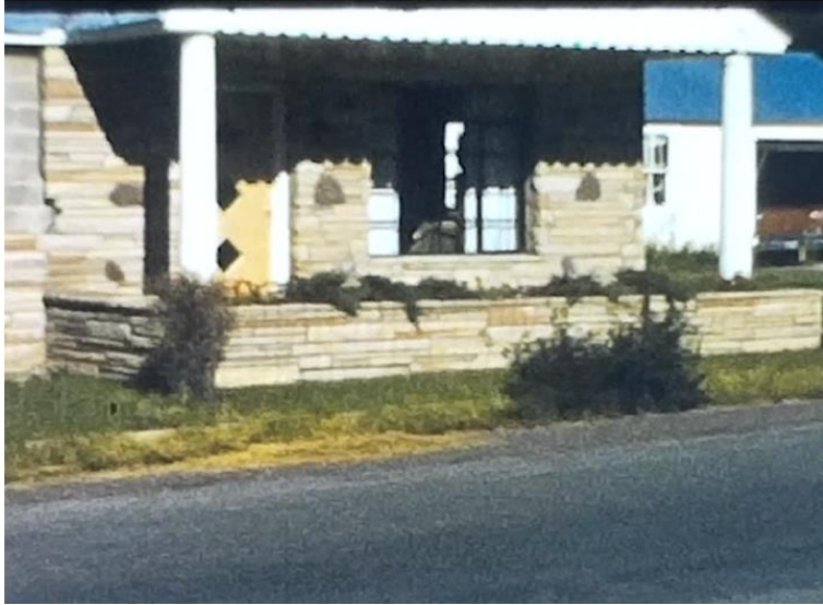
Front porch, facing east.
