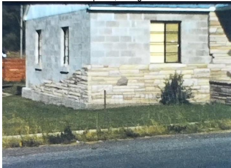
Northwest Oblique (northern half of front [west] façade)
