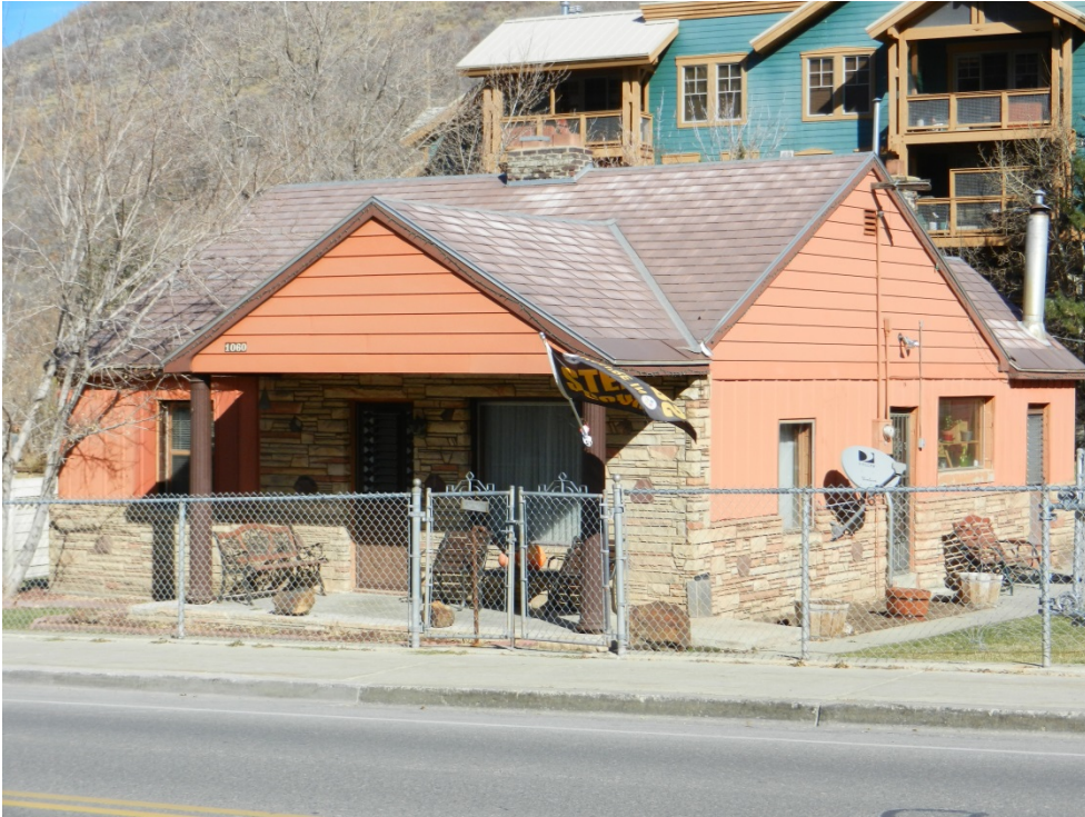
1060 Park Avenue. Southwest oblique. November 2013.
