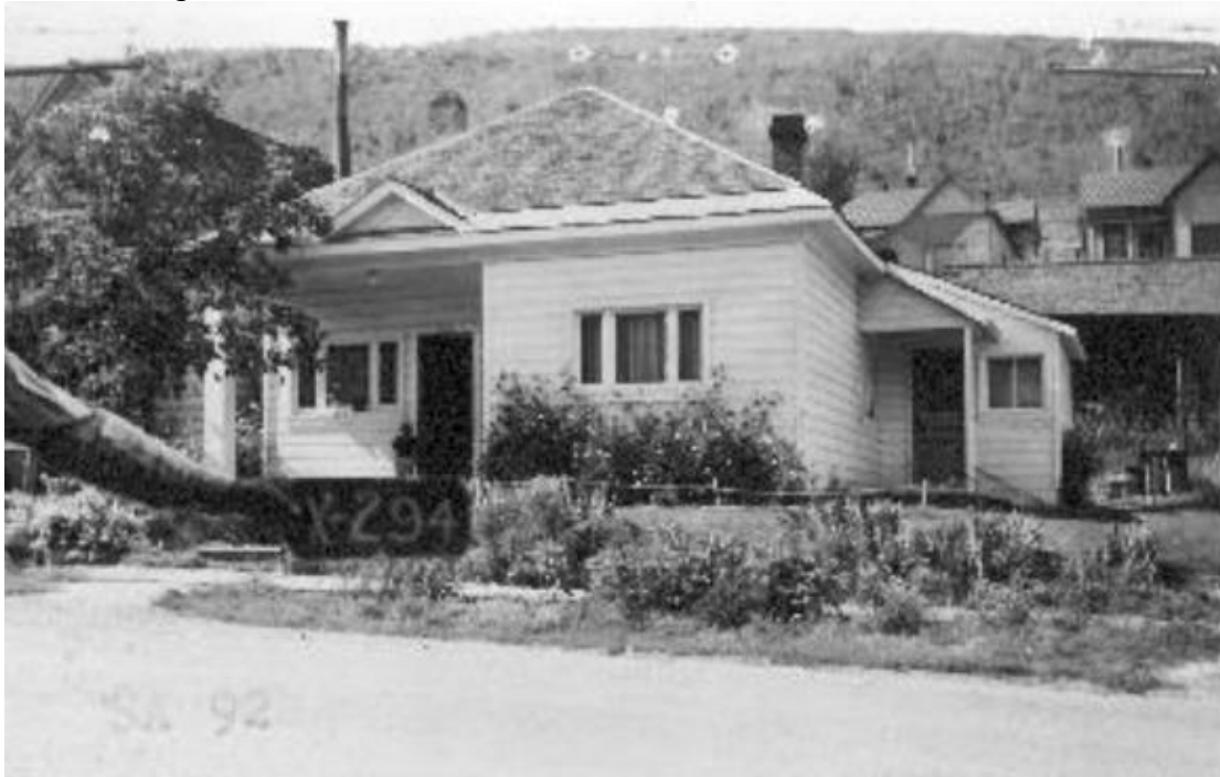
Figure 2: 1057 Woodside Avenue circ. 1940 tax photograph. Visible in this photograph are the circ. 1918 alterations, the circ. 1936 north addition, and the corner of the outbuildings.
