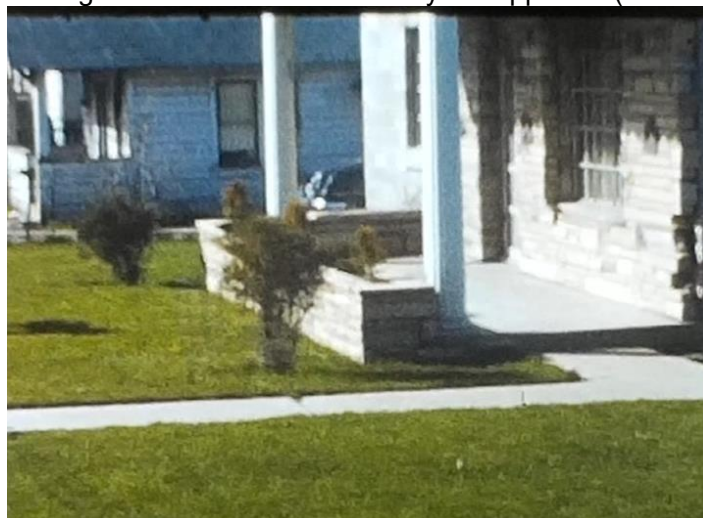
Front porch facing north.
