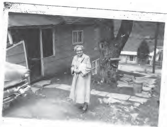
C.1950 photorgraph showing the wood shed on the left side of the porch.
