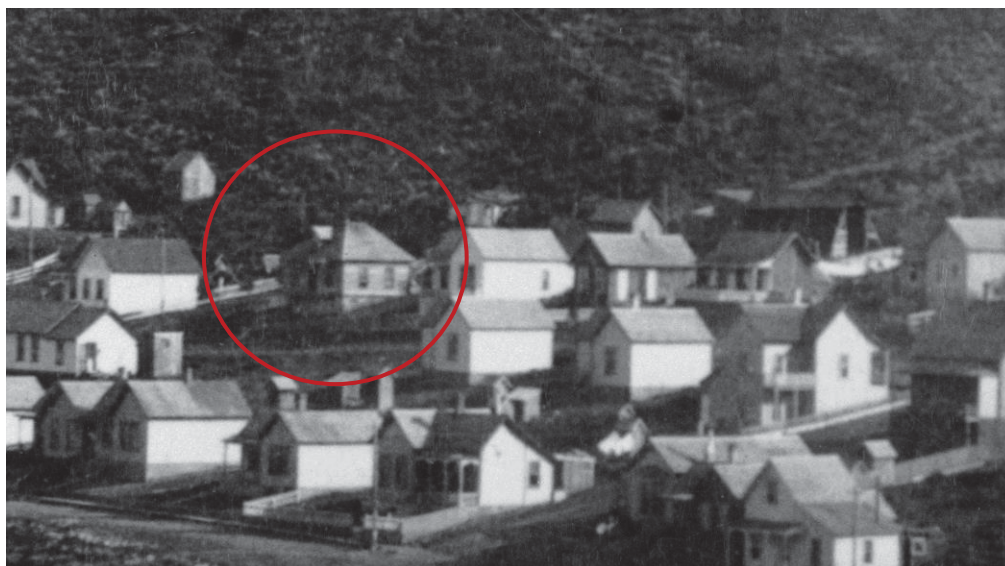
This c. 1900 photograph shows the basement addition, but not the rear addition. Photo courtesy of the Utah State Historical Society.
