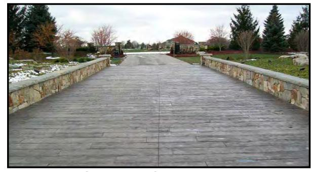
'Wood' Stamped Concrete for Bridge Element
