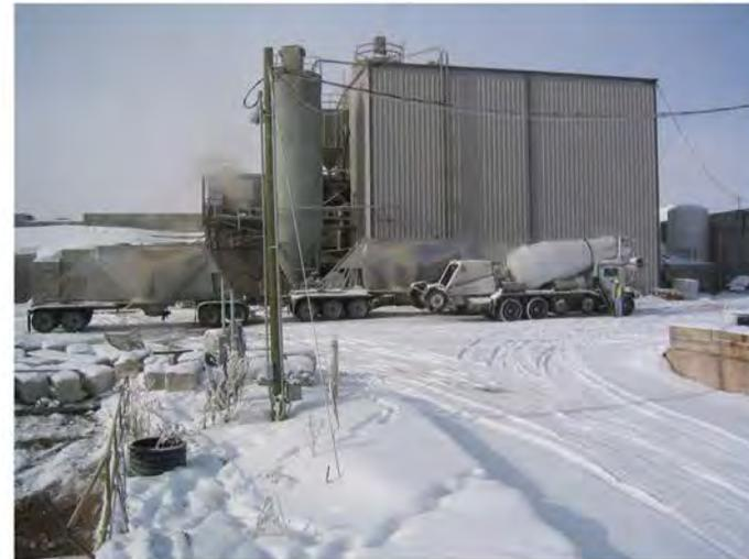
Bulk cement delivery, sand and gravel delivery trucks are 50 feet long, and with pup are 85 feet long, versus concrete mixer trucks which are 34 feet long. Batch plant building and silos approximately 40 feet high.
