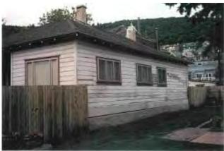
This photograph of the north side elevation shows the Chicago-style windows that had been installed in the 1920s. The ghost lines remain of the original double-hung windows that would have been used on the earlier cross-wing.
