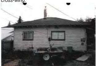
These photographs of the west (rear) elevation of the house shows that the addition extended the hipped roof form that was added in the 1920s, rather than adding a new roof form to the existing form. Note that there are no breaks in the roof form, though we know from the tax cards that this rear addition did not appear until 1941-1968.
