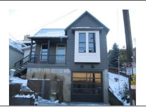
Though this house at 1063 Norfolk Avenue is historic, it is a good example of how the important it is to maintain existing grade as much as possible. The steel retaining walls were meant to help ground the historic house with plantings that would shield the foundation; however, the retaining walls have become a dominant site feature.
