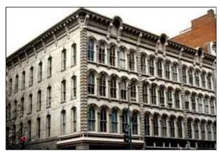
The historic cornice was successfully replaced with a The surfaces of substitute materials may fiberglass cornice. Photo: NPS files.
