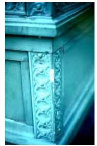
Substitute materials need to be located with care to avoid damage. The fiberglass column base has chipped, whereas the historic cast iron would have remained sound. Photo: NPS files.
