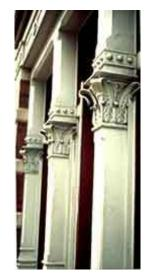
Cast aluminum has been used as a replacement material for cast iron. Photo: NPS files.
