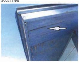
Loose and damaged soffit
