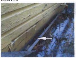
Siding in contact with the ground
