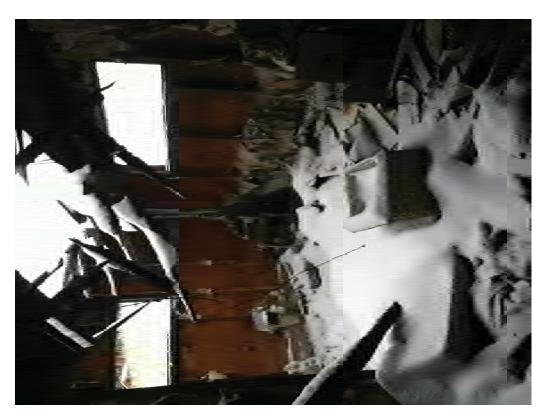
Fire-damaged rear addition. Note the horizontal lumber atop vertical studs.
