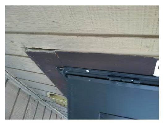
Original wood trim. Note the reveal. Layers of Bricktex and vertical wood siding have hidden much of the reveal on this original trim.
