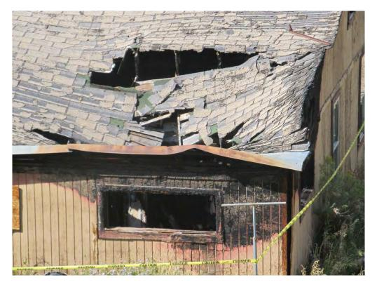
Fire Damage on South Elevation
