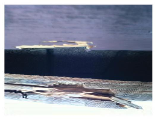
Bricktex beneath vertical wood siding. The original wood lap siding is likely beneath this layer of Bricktex.
