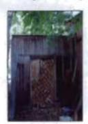
The first floor of the original hall-parlor house is obscured by later additions, but it should be noted (see plans) that some of the original drop-novelty wood siding is extant on the west wall of the house. It has been covered with wallpaper and additional materials and is not completely visible. Remnants of roofing tar along the upper section of the west wall show that the original shed roof met the house at a higher elevation.
