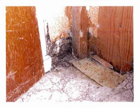
STRUCTURAL SYSTEM. Interior flooring settlement/wood rot.
