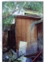
Addition 2: The wall is clad in T1-11 with a narrow exposure between vertical channels. Centered in the rear façade is a two-angle bay window with fixed sidelights and paired central three-over-three awning type windows. The window was badly built, is in terrible disrepair, and has no salvage value.
