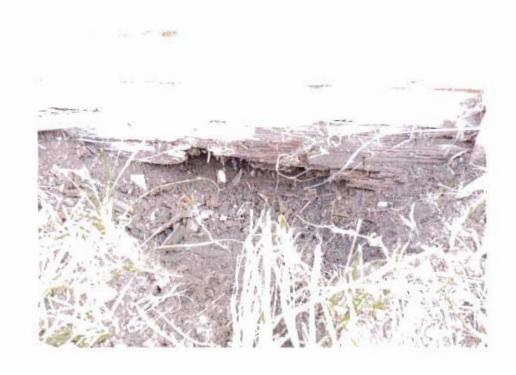
**FOUNDATION**. Rotted sill plate on south side sitting on bare earth (no foundation).
