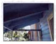
Front porch: A 2/12 pitch partial width shed roof projects from a 2"x10" ledger board attached to the exterior siding of the primary façade.
