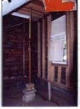
where the original footing and/or foundation material was removed. The front and south sides of the building are suspended above the bottom of the trench by a series of 4 to 5 pipe jacks located haphazardly on the interior dirt where the floor joists and decking have been removed.
