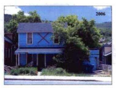
The horizontal drop-novelty siding on the first story is approximately a 6 %" exposure. The second story also has a horizontal siding with a 6 %" exposure but it is a tongue and groove type. Both are original but are severely weathered and checked; some boards are cracked their full length. The 1" x 4"
