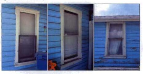
on all three facades of addition 2. There is no evidence to suggest these windows were once part of the original house and could not be reused because they are in severely deteriorated condition.
