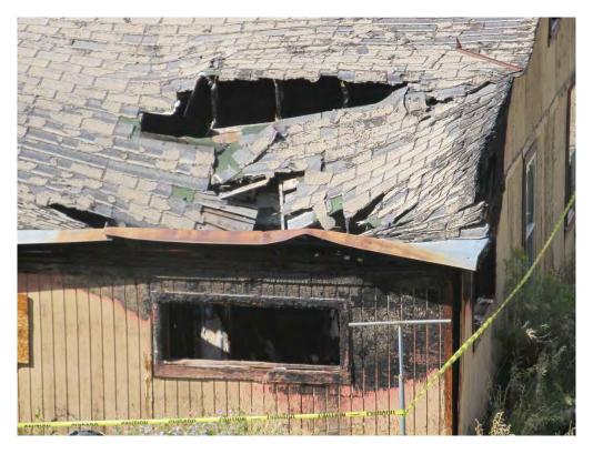
Fire Damage on South Elevation
