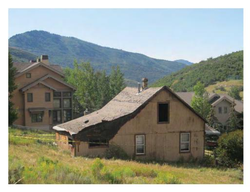
East Elevation (note fire damage)
