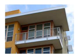
A Balcony is a private personal open space providing access to light and air above the ground level. Metal or slab balconies may project out from the building face, be semi-recessed, or completely recessed. Balconies must be surrounded by guard rails or a building face. A balcony typically has French or sliding glass doors leading out onto it and can be entered from a living room or bedroom.
